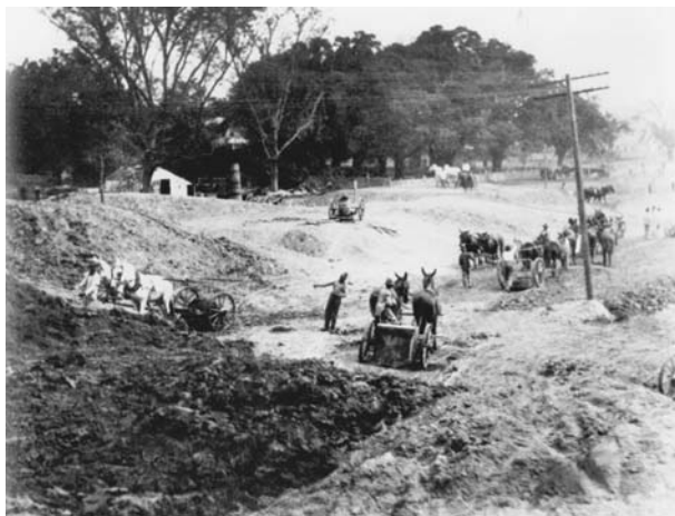
Figure 11: Material is delivered to an early levee construction on the Mississippi River (circa 1860–1925)
