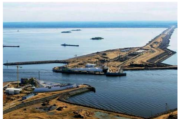
Multisector funding – St Petersburg's integrated flood defence and highway project
