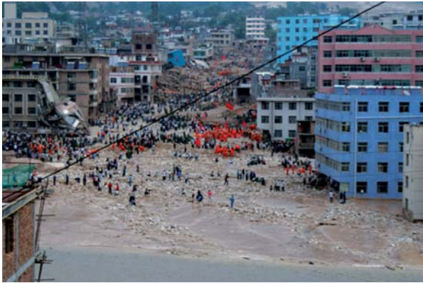
Figure 91: Buildings in Zhouqu City surrounded by mud as rescuers attempt to locate missing persons
