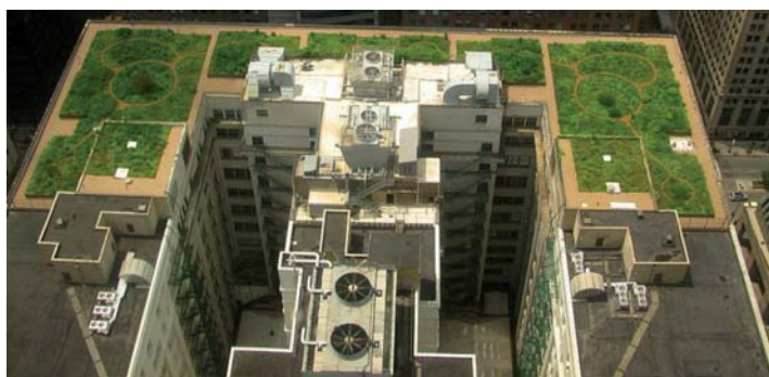
Chicago's City Hall building – the first municipal building in the United States to host a green roof
