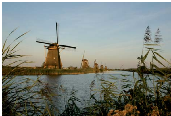
Figure 10: A windmill lifts water to channelized rivers that carry water at a high level above the floodplain to the coast ; typical in the Netherlands and England
