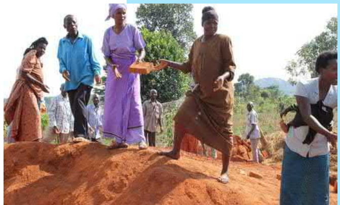
Laying bricks for construction of the storage tank
