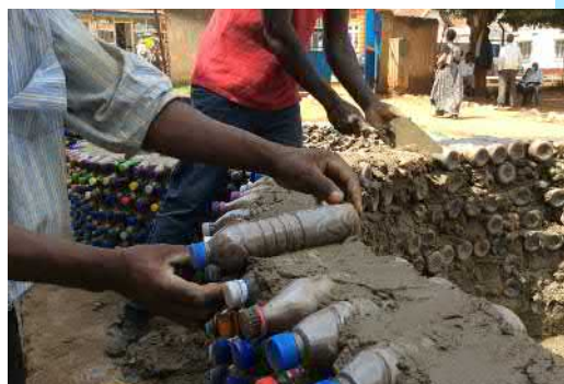
Plastic bottles being used as bricks for the water tank
