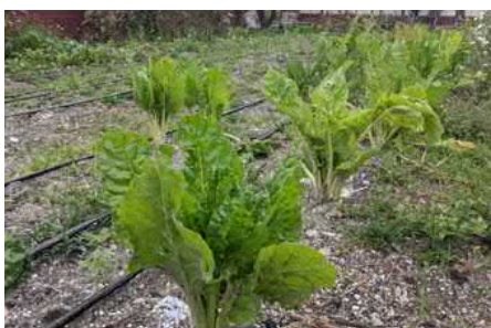
Irrigation system for the school garden
