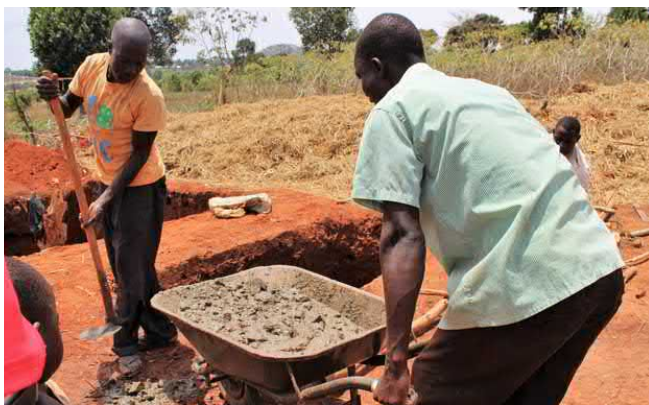
Mixing concrete for construction of the storage tank
