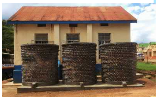
Completed tanks made from recycled plastic bottles
